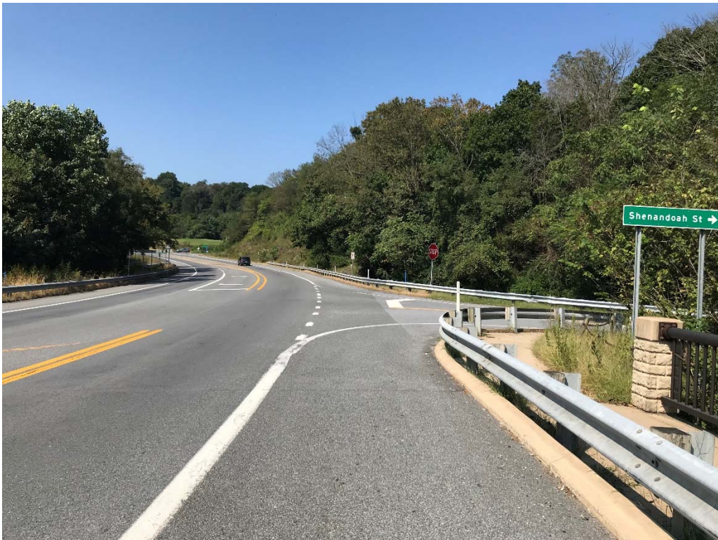
US 340 Southbound Approach to Shenandoah Street
