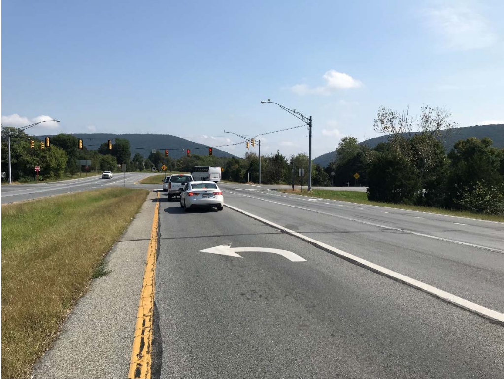
US 340 Northbound Approach to Washington Street/Shoreline Drive
