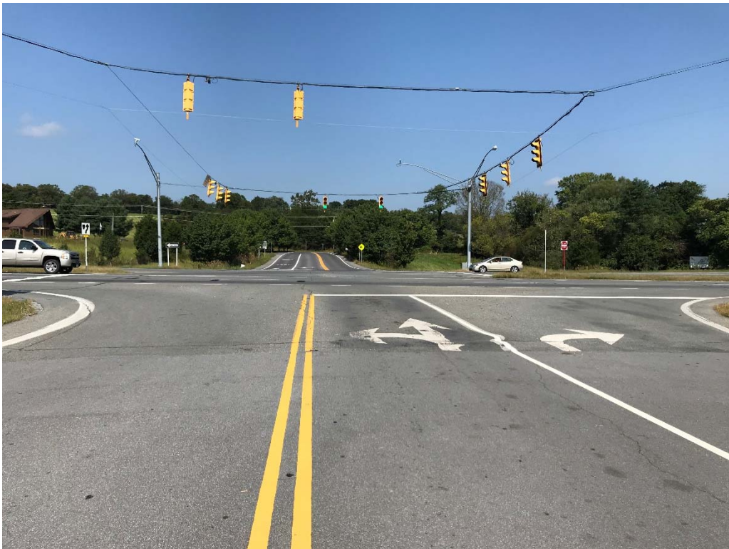
Shoreline Drive Westbound Approach to US 340
