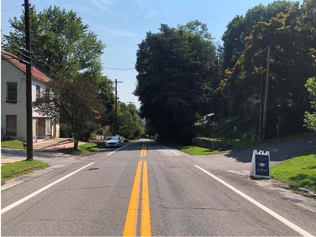
Washington Street Eastbound Approach to Columbia Street
