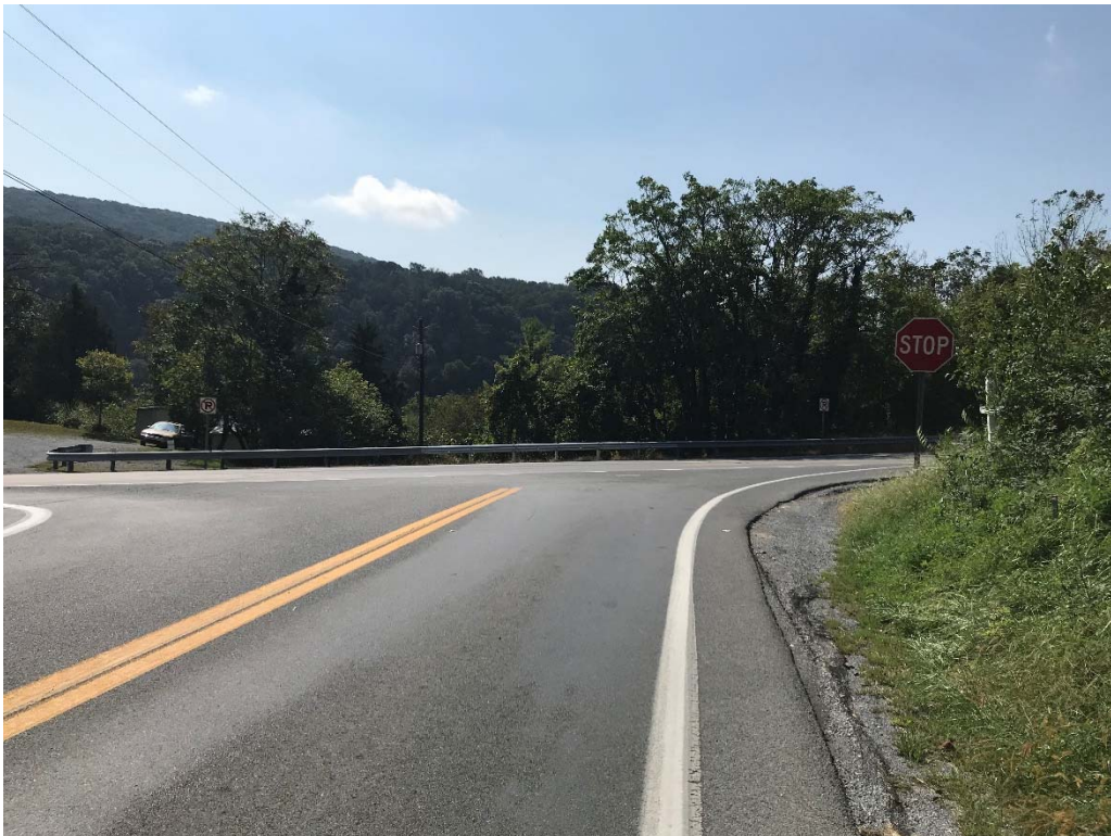
Union Street Eastbound Approach to US 340
