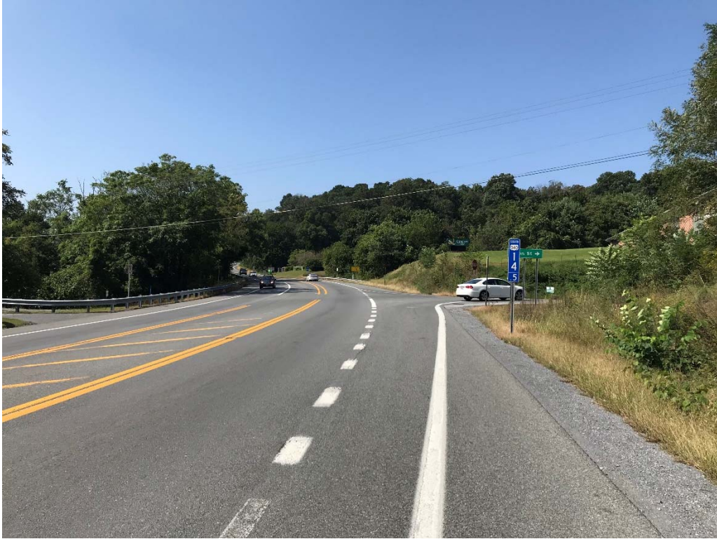
US 340 Southbound Approach to Union Street
